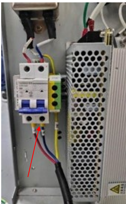
Figure 22.16: Main power to generator
